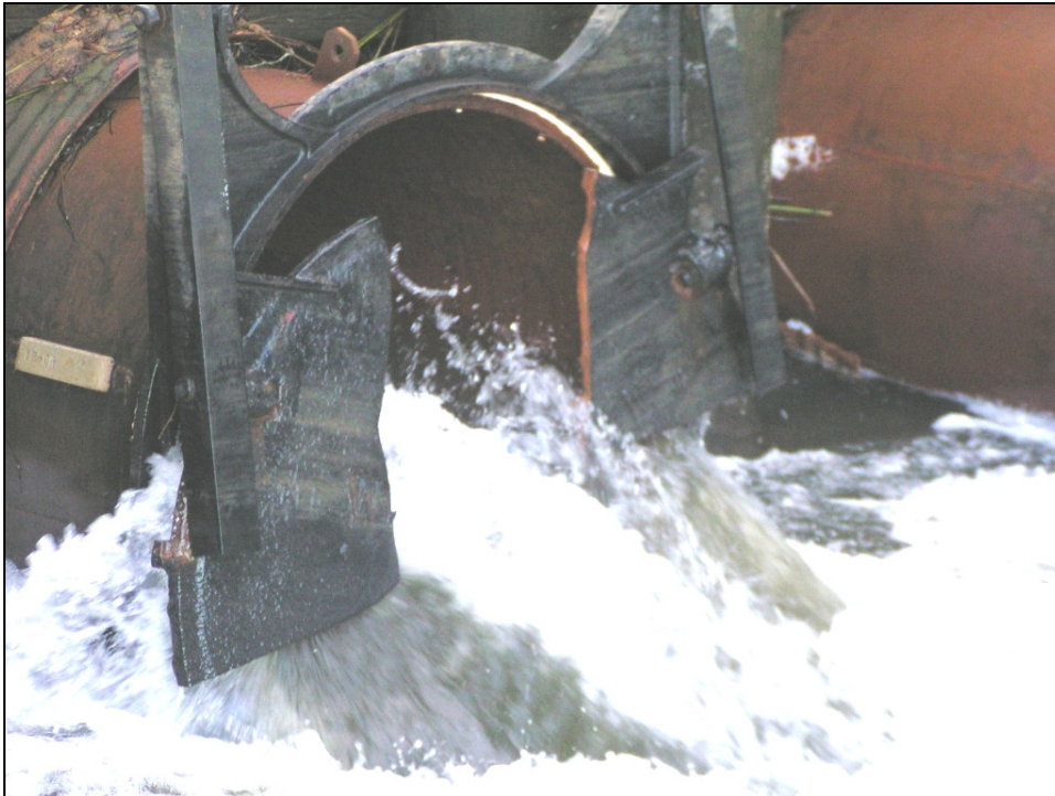
Photo 1 - Broken 60" flap gate
